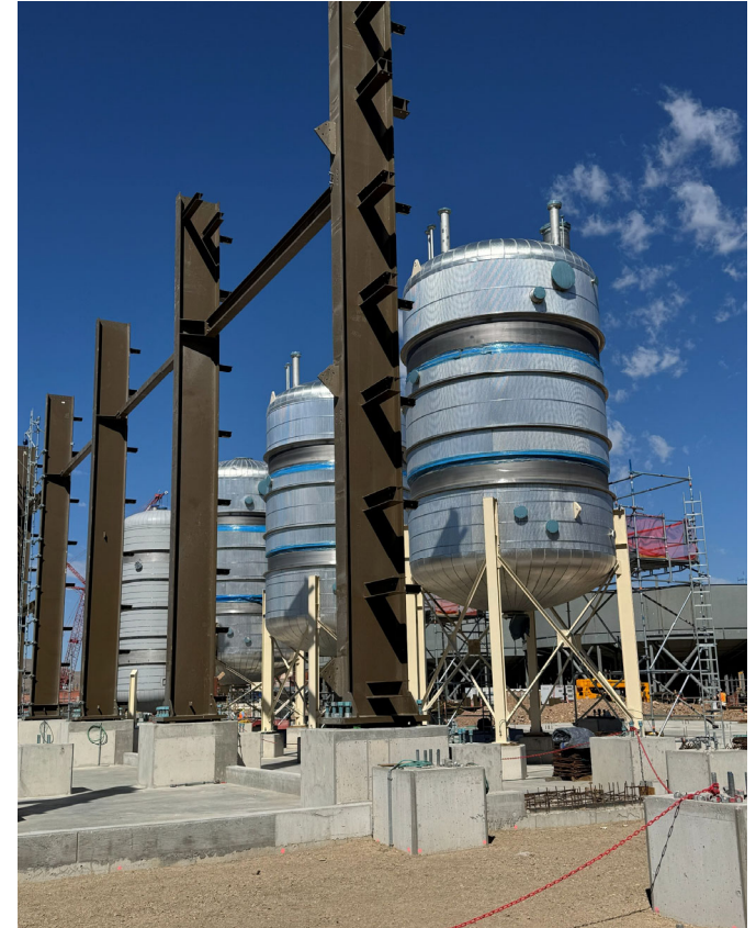
Steel structure erected for the Lithium Carbonate Crystallization facility adjacent to the bicarbonate reactors
