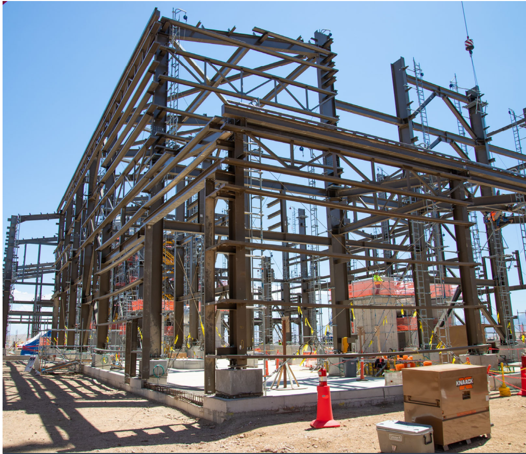
Progress at the Magnesium Sulfate building
