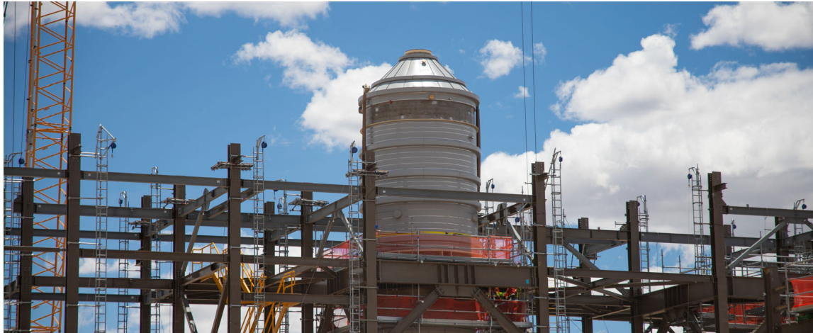
The first crystallizer has been installed in the Magnesium Sulfate Building
