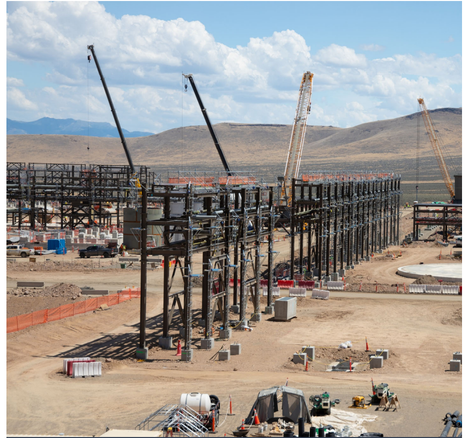
Progress on the north-south pipe rack that will connect the ROM to the main process plant
