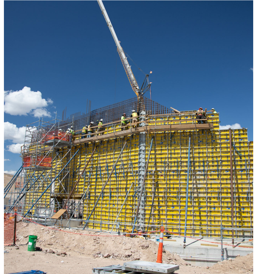
Pumping concrete into formwork for a ROM feeder breaker retaining wall
