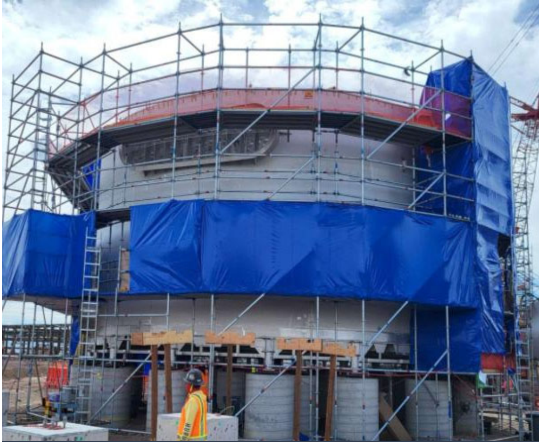
The Sulfuric Acid Plant's stainless-steel converter installation
